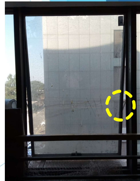
Window 41: Open Window was difficult to pull back for locking. Hinges Replaced & Restrictor Arms Installed
