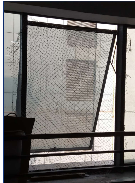
Window 41: Open Window was difficult to pull back for locking. Hinges Replaced & Restrictor Arms Installed
