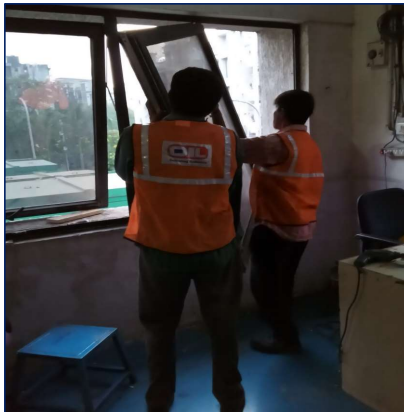
Window 1070 converted from Fixed Glass to Openable
