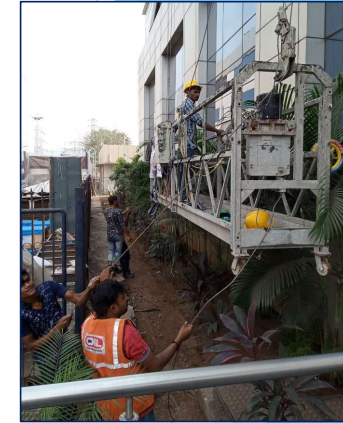
Pulling Cradle to Jump to required Level to Save Trees
