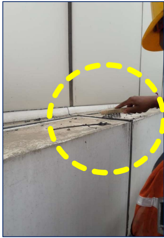
1. Removal of Existing Sealant by Blade, Wire Brush & Cleaning the debris
