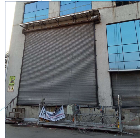
Fabrication and Installation of Aluminium Sheet above Shutter (By others)
