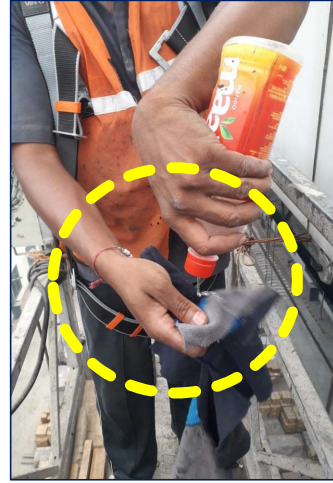
4. Surface preparation by cleaning with a solution and a cloth
