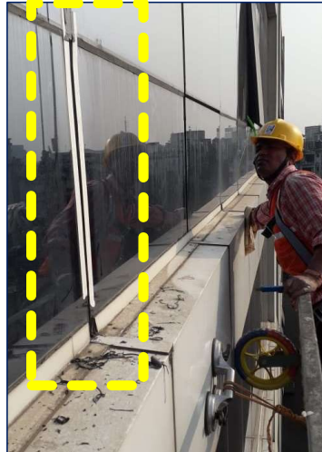
4. Surface preparation by cleaning with a solution and a cloth
