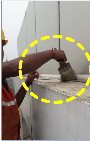
1. Removal of Existing Sealant by Blade, Wire Brush & Cleaning the debris
