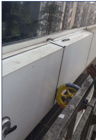
Pulling Cradle to Jump to required Level to avoid Clash with Structure
