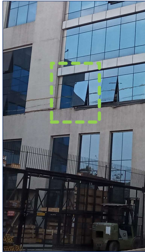
Window 1507 (After Glass Replacement)
