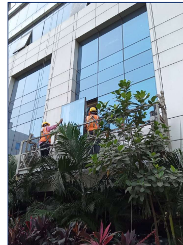
Pulling Cradle to Jump to required Level to avoid Clash with Structure
