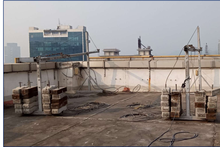
Gandola Members Assembly at Terrace Having 1000 Kg Counterweight
