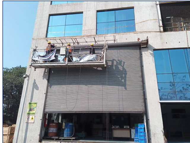
Fabrication and Installation of Aluminium Sheet above Shutter (By others)
