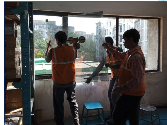
Window 1072 Installation of Glass to convert Panel from Openable to Fixed.
