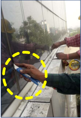
1. Removal of Existing Sealant by Blade, Wire Brush & Cleaning the debris
