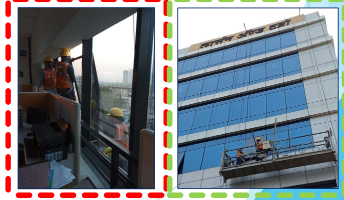
Window 238 at Office: Re-installed. Panel was shifted Down by 5mm approx.
