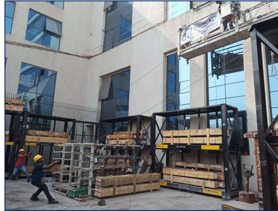
Pulling Cradle to Jump to required Level to avoid Clash with Structure
