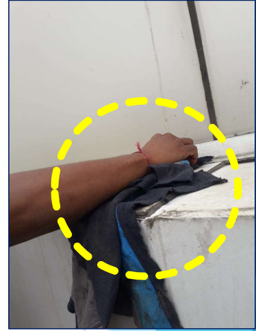
4. Surface preparation by cleaning with a solution and a cloth
