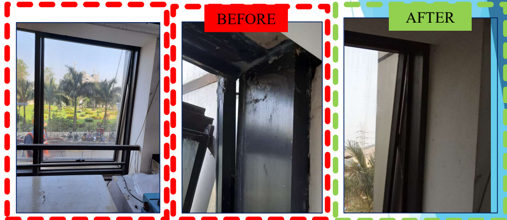
Window 382 : Frame Dislodged. Window-Reinstalled and Restrictor Arms installed.
